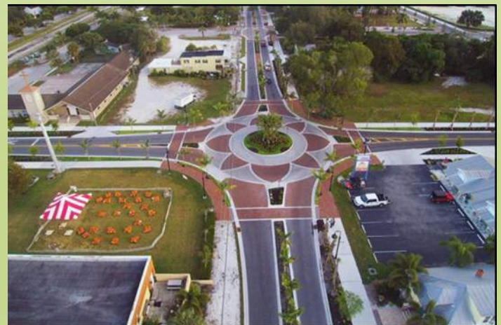
Pennsylvania Avenue/Ragsdale Street Roundabout - After
